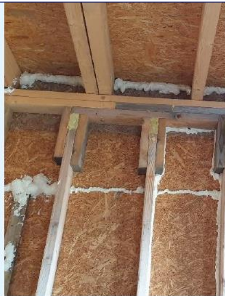
figuur 9: PUR in HSB wand in naden
